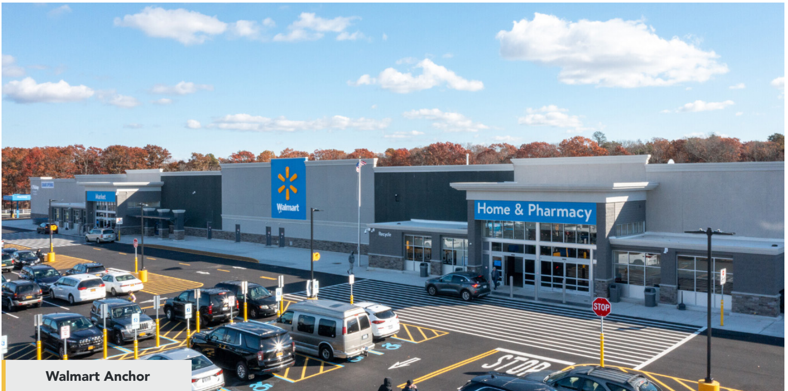
Walmart Anchor & Pad Buildings
