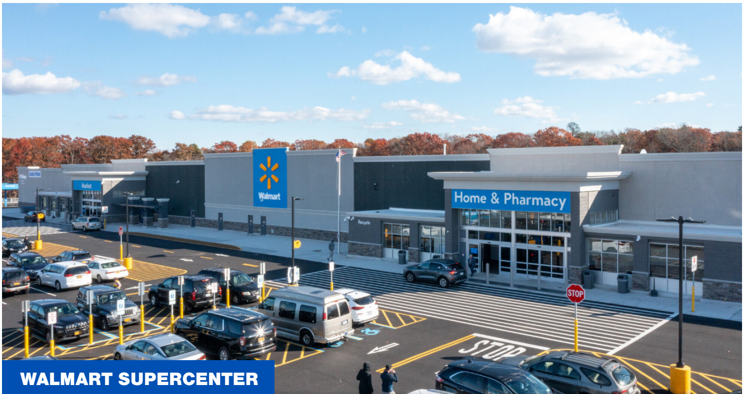
WALMART & PAD BUILDINGS
